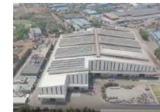
SMS INDIA Metal shed rooftop on-grid ODISHA 1700 kWp
