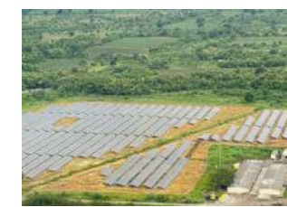
RCCPL PRIVATE LIMITED Ground Mounted In Premise BTM MAHARASHTRA 5.0 MWp
