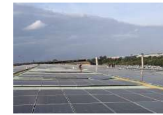
JINDAL ALUMINIUM Metal Shed Rooftop Behind the Meter KARNATAKA 6.0 MWp
